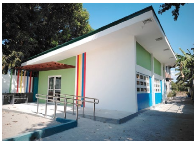
The CDC in Barangay San Jose South, Anao, Tarlac is among the eight CDCs recently constructed using funding assistance from the national government. It was completed on April 29, 2026.
