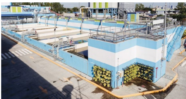
The Poblacion WTP treats 150 MLD of water from the Laguna Lake and supplies water to around one million customers in Parañaque, Las Piñas, Muntinlupa, and Cavite. It was inaugurated by the President on December 15, 2023.
