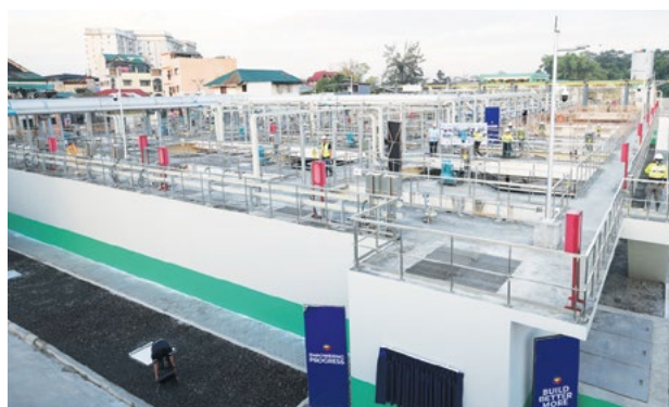
The 60-MLD Aglipay Sewage Treatment Plant in Mandaluyong City treats the domestic wastewater of over 650,000 Manila Water customers. It was inaugurated by the President on January 16, 2026.
